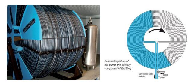
**Figure 4.** Biosling system. Coils of plastic hoses constitute the main component. The photo shows eight coils working in parallel. The vessel shown in the background accumulates the upgraded gas and separates it from water saturated by carbon dioxide (Courtesy: Artic Nova, Sweden).
