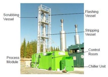
**Figure 9.** Biogas upgrading unit at Motala (unit supplied by Greenlane® Manuka - 80 Nm3 hour<sup>-1</sup> capacity; Source:www.flotech.com)
