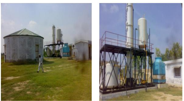
Figure 16. Biogas plant (left) and upgrading unit (right)
