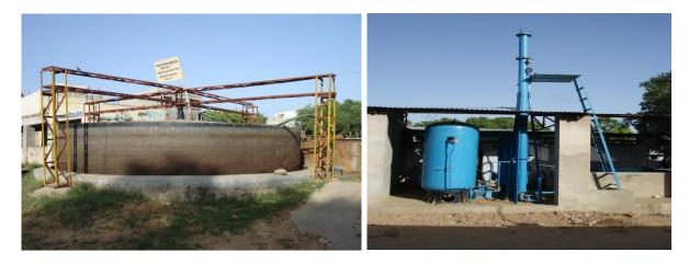
**Figure 12**. Biogas plant (left) and upgrading unit (right) (Source: Prof. V.K.Vijay, IIT Delhi, India)
